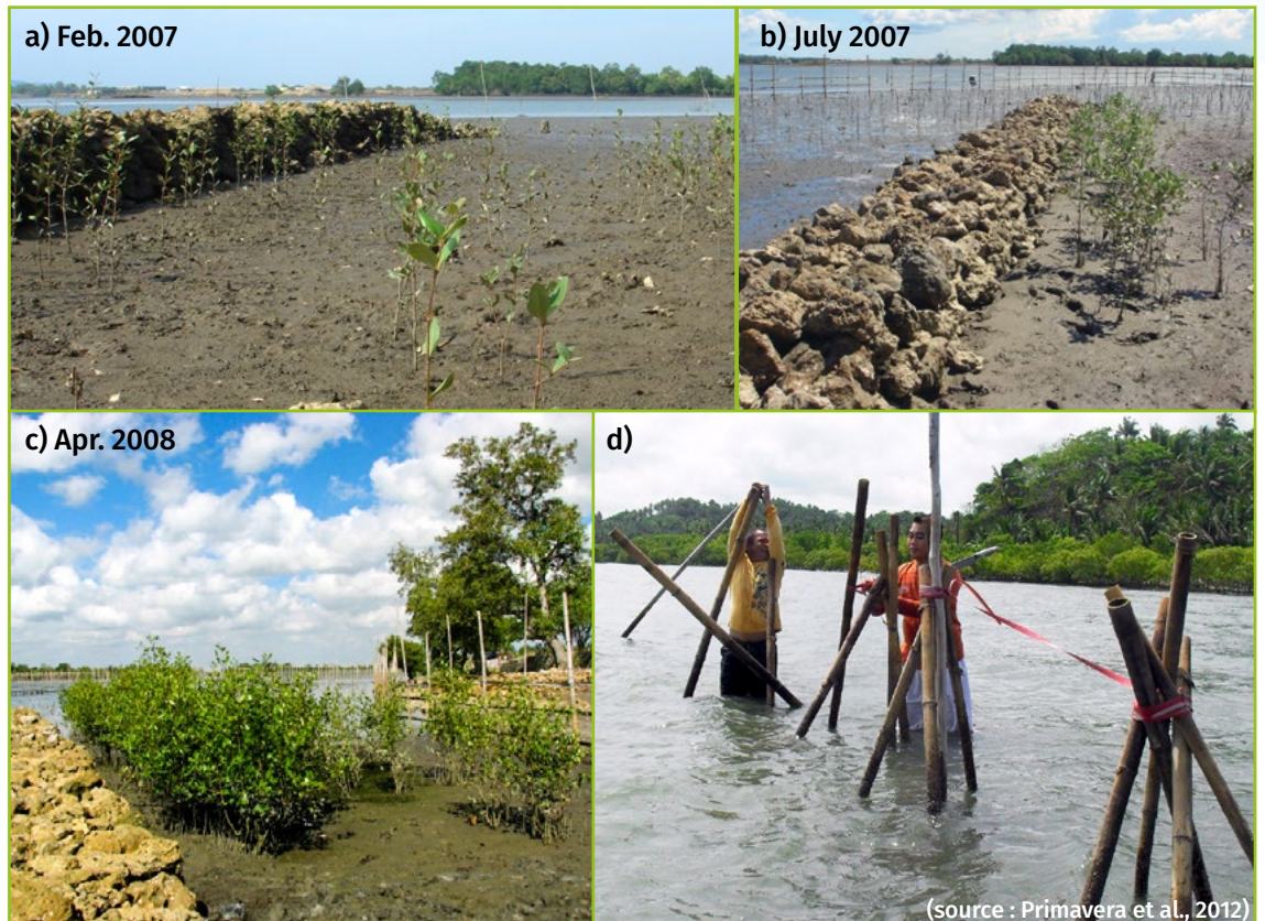
Figure 5 5 Photos A, B, and C: walls used as breakwaters: rapid mangrove growth is evident within one year. Photo D: bamboo structures to disperse wave energy.
