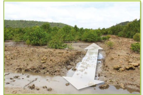
Figure 9 Example of the creation of a breach in a human-modified mangrove area using an excavator. This operation resulted in subsequent natural colonisation of the area behind the topographic feature: 6 different species flourish there! (source : Lewis & Brown, 2014)
