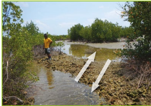
Figure 8 The dyke is high enough to prevent drainage of the water body in the background. A hydrological reconnection is required. (source : modified d'après Lewis & Brown, 2014)
